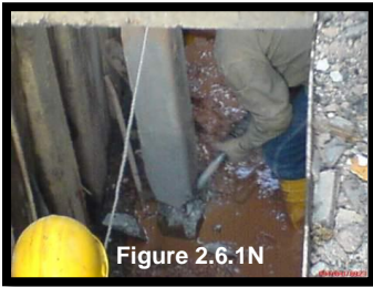
Hacking off unwanted piles to cut-off level
