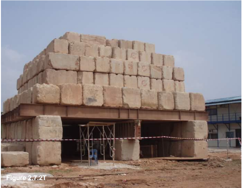
Pile Testing in progress
