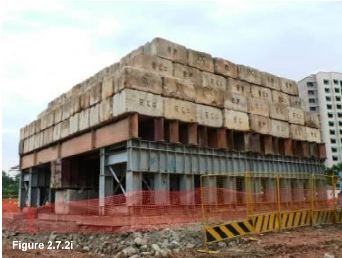
Completed set-up of pile load test
