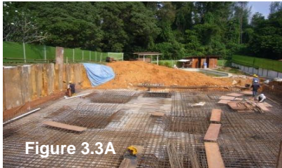
Figure 3.3A Basement raft construction in progress
